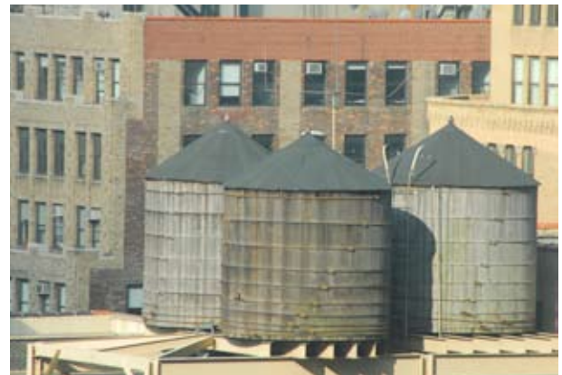
Wooden New York roof top tanks
